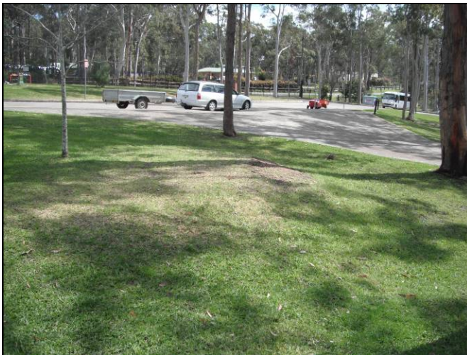
Figure 7: Possible mound of surficial filling in south-western area of site
