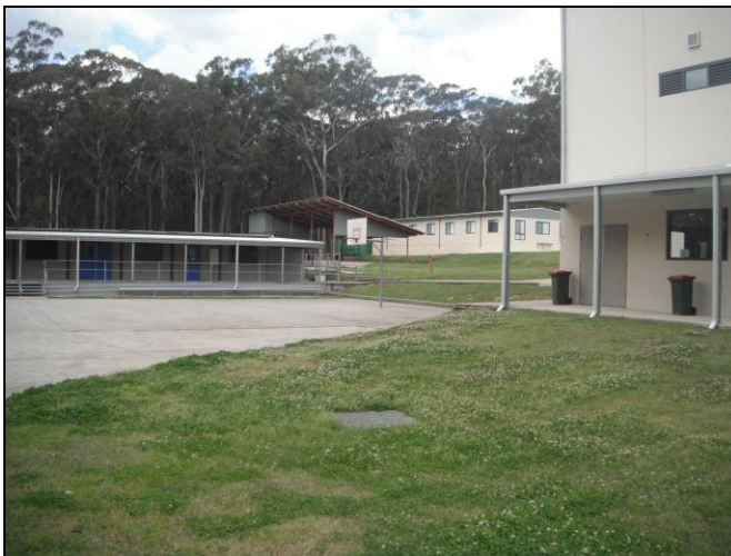
Figure 2: View of existing building, looking south-west
