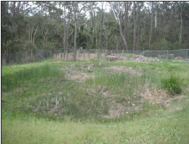
Figure 8: Detention pond in north-east corner of school grounds
